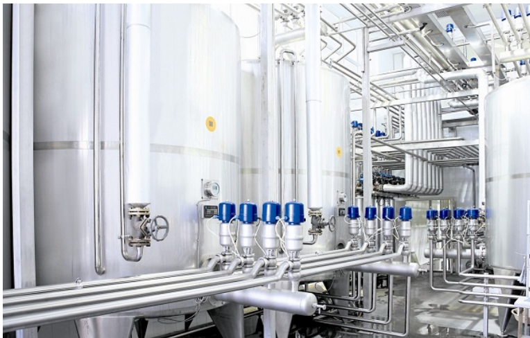
Figure 3 CIP System - Piping Reference Image
